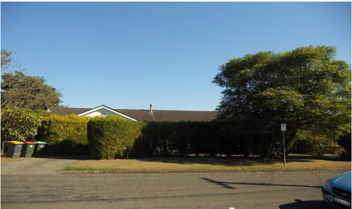
Figure 19 - View South Towards 20 Garthowen Crescent
