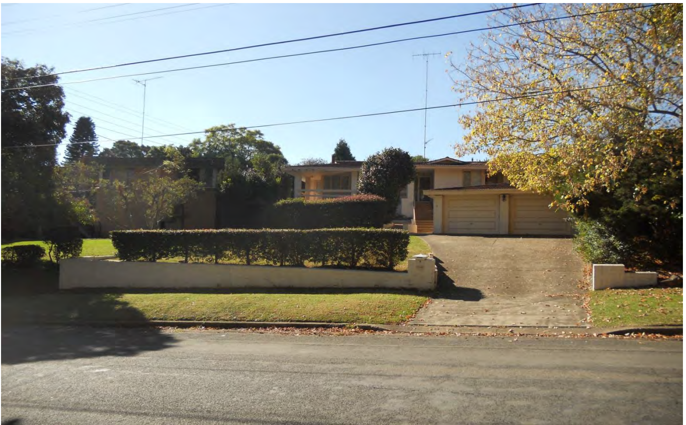
Figure 7 - View North Towards 6 Garthowen Crescent
