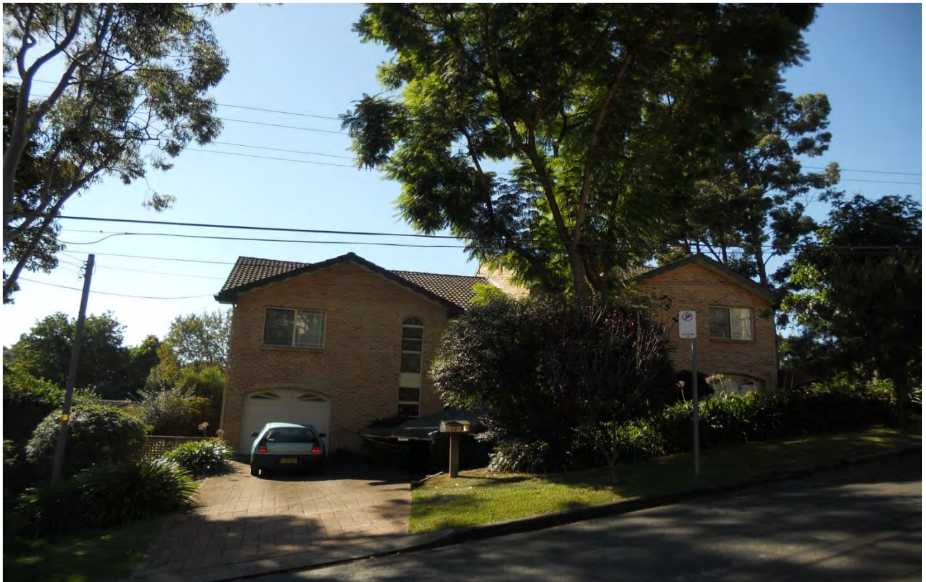
Figure 10 - View North Towards (Duplex) 12 Garthowen Crescent
