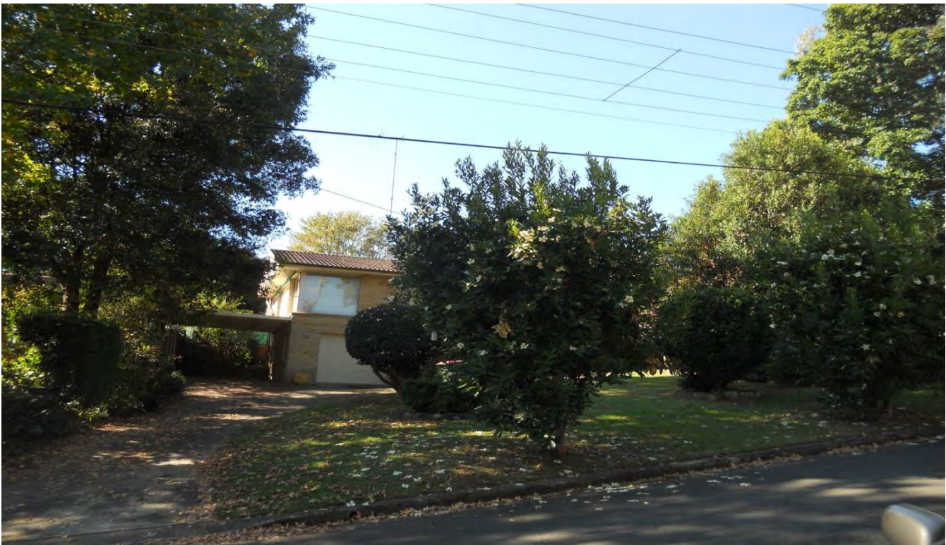
Figure 9 - View North Towards 10 Garthowen Crescent
