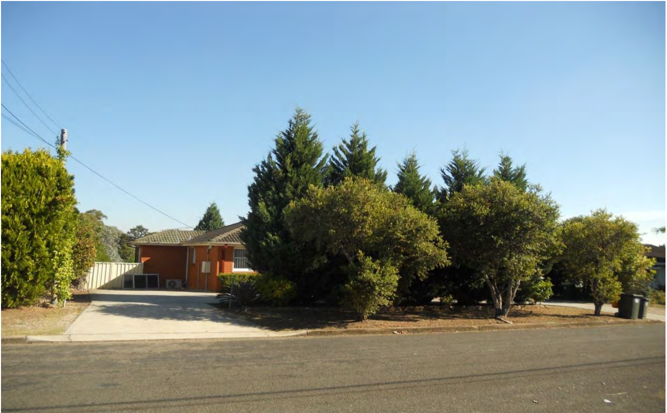
Figure 20 - View South Towards 22 Garthowen Crescent
