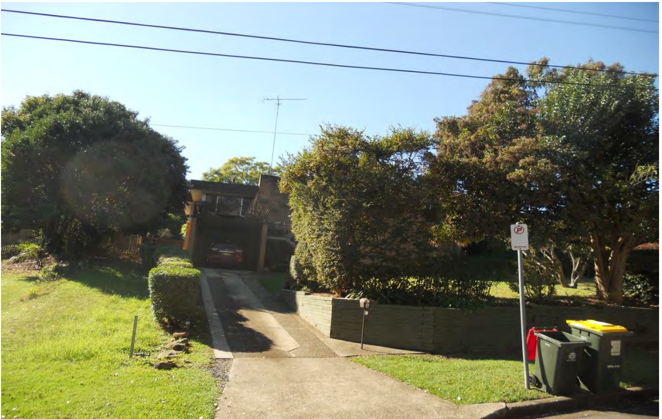
Figure 6 - View North Towards 4 Garthowen Crescent
