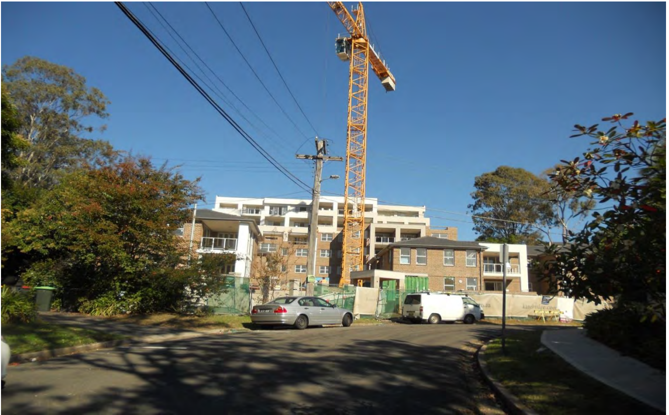
Figure 23 - View East Towards New High Rise RFB's in Garthowen Crescent
